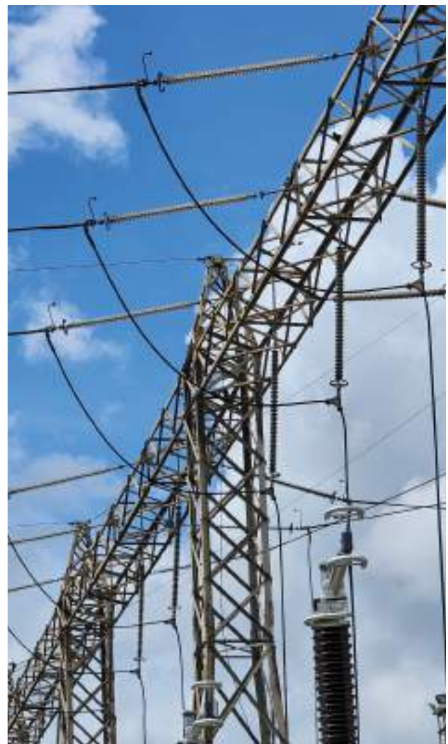
Polymer based insulation in Transmission Tower at Surat
