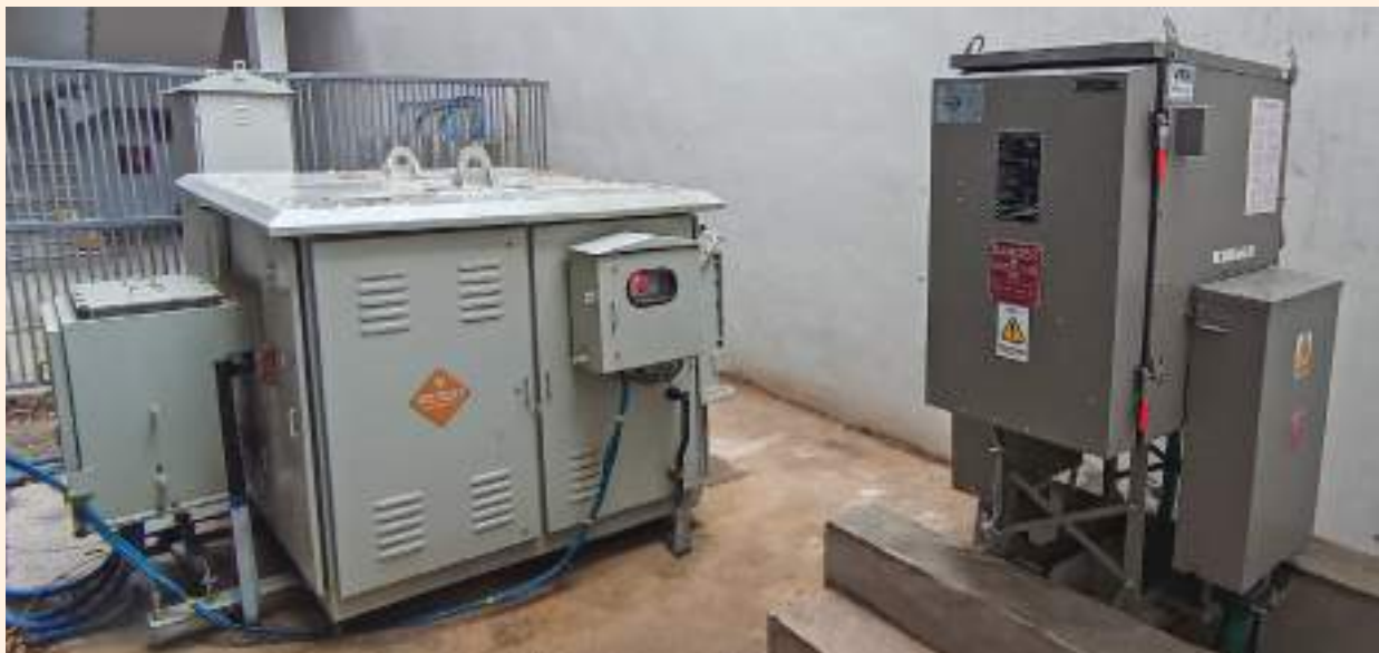
Distribution Transformer at Agra
